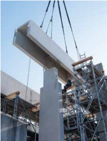
New beams of the Great Hall at the Museum of Anthropology at UBC being installed in February 2023. (Photo: Michael Elkan)
