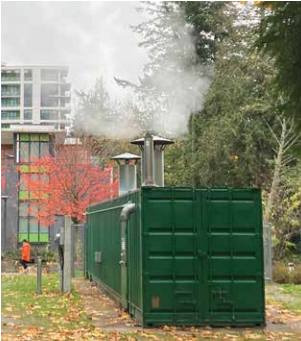
One of two energy centres in the Neighbourhood District Energy System, located along the South Campus Greenway near the entrance of UBC Farm. Both energy centres heat water and distribute it to residences in Wesbrook Place through a network of underground pipes. (Photo: Eagle Glassheim).
